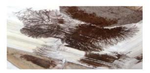
The most common form of wet rot is the cellar fungus (Coniophora puteana). This is associated with timbers in constant contact with damp conditions; such as lintels, skirting boards and floor joist ends. Cuboidal cracking is smaller than with dry rot fungus and adopts a darker appearance. The mycelium of the cellar fungus is fern shaped and will vary from dark brown to black. There are many types of wet rot they are not regarded as dangerous to the building as dry rot.
