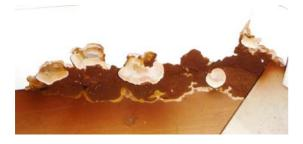
Where there is a fruiting body or sporophore of the dry rot fungus, a red dust will appear; these are the spores of the fungus. These spores are microscopic and there will be millions of spores present during a virulent attack of dry rot fungus. Dry rot spores can be found in most buildings although no germination will take place as long as conditions within the building remain dry. Other types of brown rots commonly encountered within buildings are known as the wet rots.
